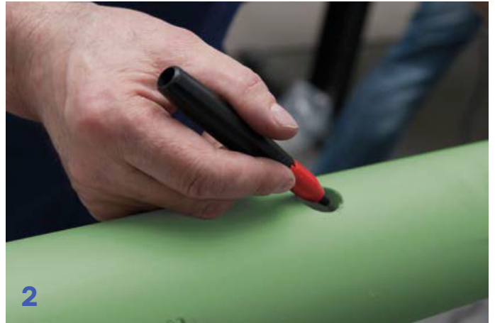
2. Processing the hole – removing the burrs made when drilling.
